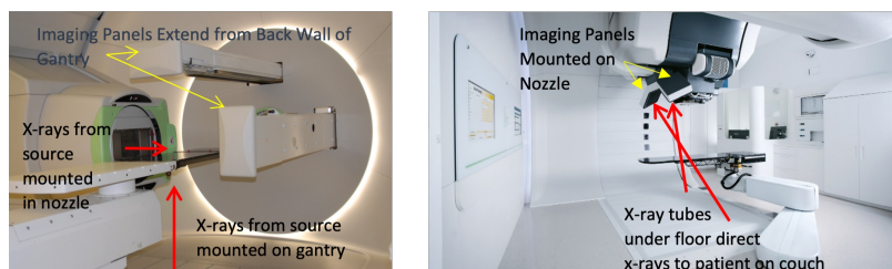
Figure 17. Two typical arrangements for the imaging equipment on the gantry.
